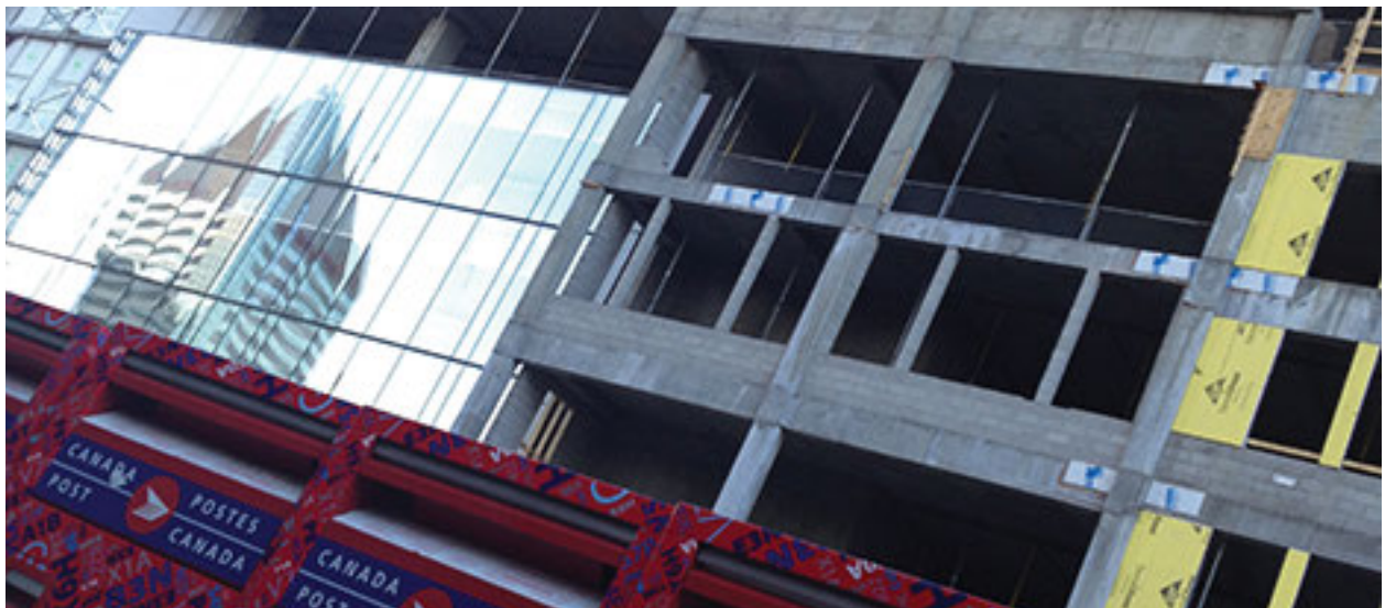
Standard Letter Boxes at Kelly Ramsey Tower in Rice Howard Way, Edmonton (Photo by L. Swaren)
